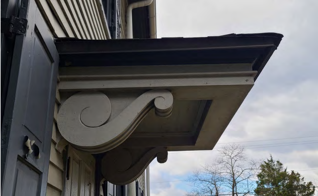
Photo E-11. Detail of the north side porch/stoop overhang showing the scroll detail that is also present over the rear entry to the enclosed south porch.
