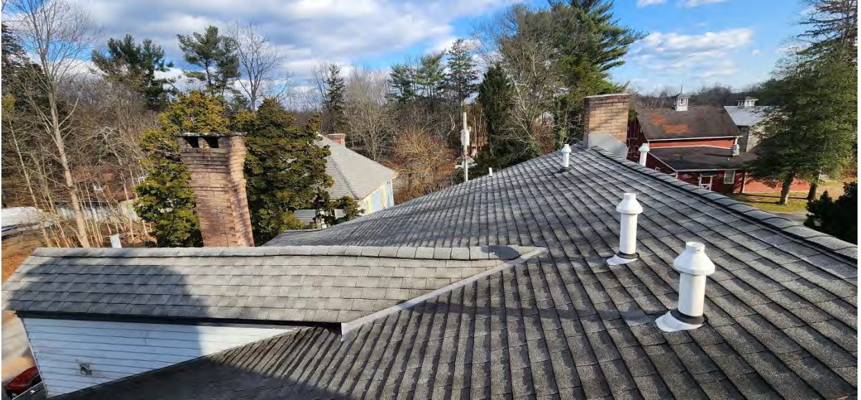
Photo E-25. Overall view of the asphalt shingle roof, which appears to be newer and in good condition overall.
