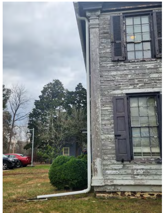
Photo E-12. Detail of the two-story pilasters at the Federal style section of the house. Note the wholesale paint loss on the siding and trim elements. Based on the manner in which the paint is peeling, the lower paint layers have failed causing the paint to check and alligator.
