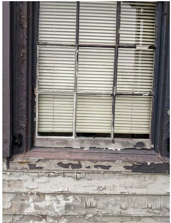
Photo E-20. Paint and glazing putty loss is prevalent at many of the wood-hung windows and frames.
