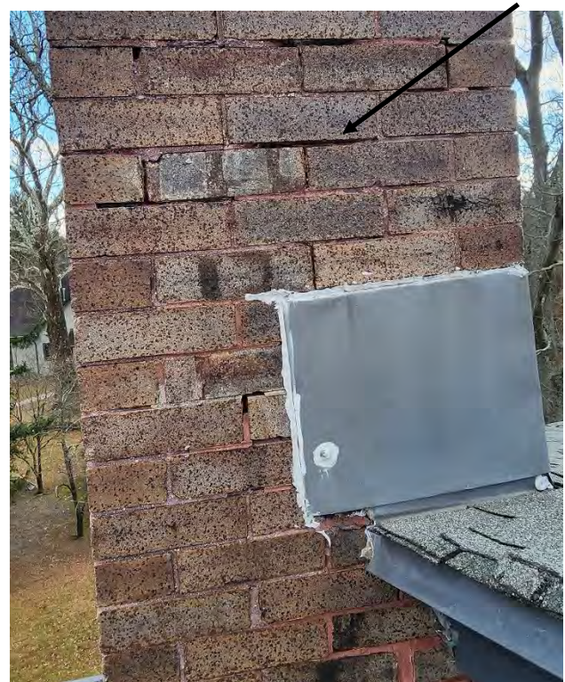
Photo E-24. View of flashings at chimney, which are generally poorly executed. Also noted in this image is mortar loss at the brick.
