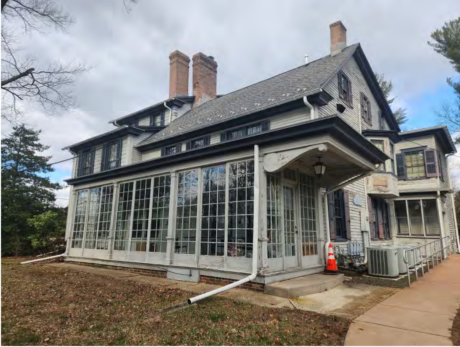
Photo S-3. View of the typical extension of the leaders to splashblocks.
