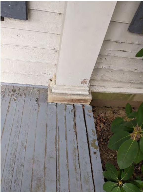
Photo E-18. View of wood rot and movement in the porch decking at the front porch.
