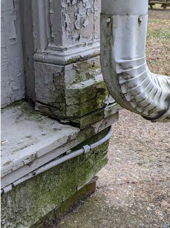
Photo E-15. Another exterior paint issue is heavy biological growth, as seen in this image probably caused by backsplash from concrete surface around the south enclosed porch.
