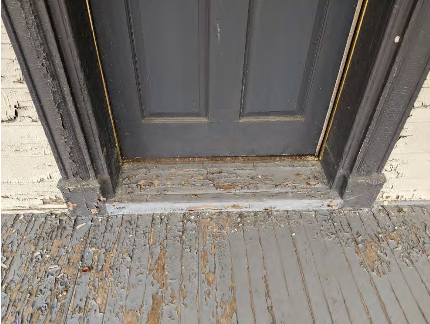
Photo E-17. View of paint failure at the front porch. Paint failure is unsightly but will also lead to wood rot and deterioration when the underlying substrate is exposed to moist and wet conditions.
