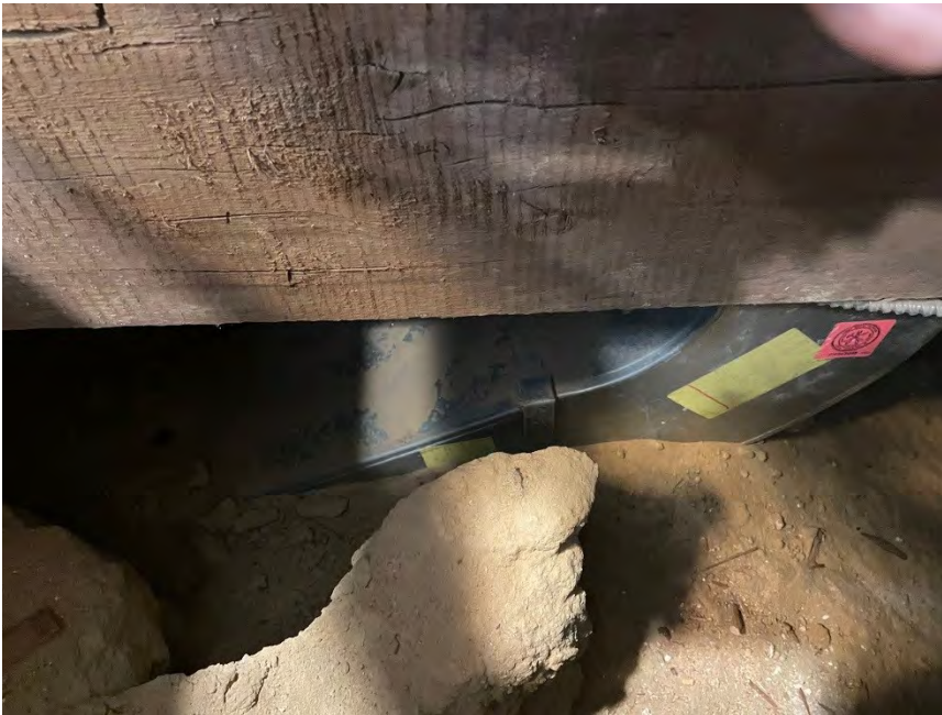
Photo I-32. View of the duct that sits close to the foundation mostly covered in sand. This sand came from underneath the fireplace supports.
