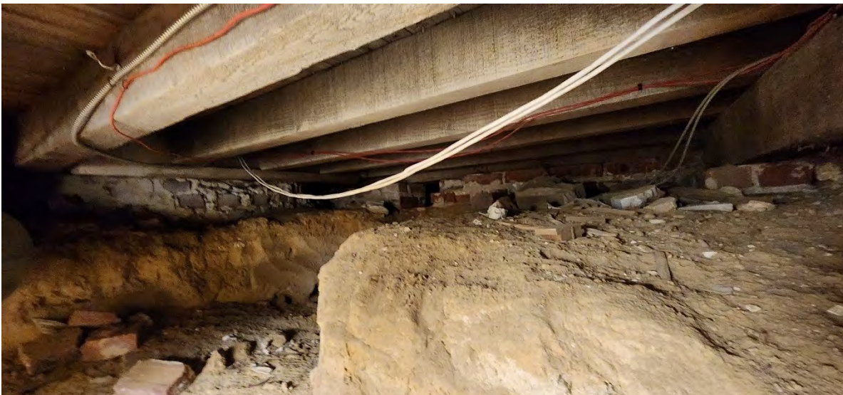
Photo I-4. View of the crawlspace looking northeast showing how portions of the crawlspace have been dug out.
