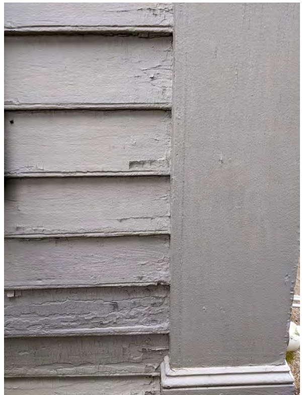
Photo E-16. This image shows heavy paint layers that were not properly sanded, and the build-up of paint is causing the paint to alligator and check.
