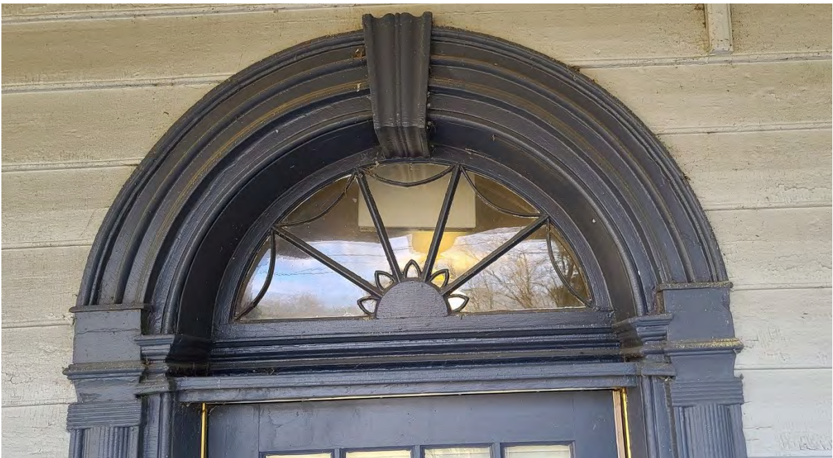
Photo E-8. Detail of the Federal style transom at the front entrance.
