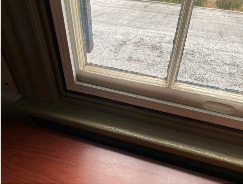
Photo I-37. View of a typical interior storm. Many of the storms were removed at the time of the condition assessment despite the cold weather. These storms are compression type with a plastic film stretched between the vinyl frame. Aluminum storms with operable glass sashes including screens may be a better option.
