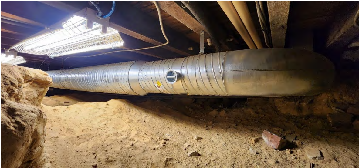
Photo I-3. View looking northwest into the north crawlspace. Note the sandy soil and the juxtaposition of the newer ductwork.
