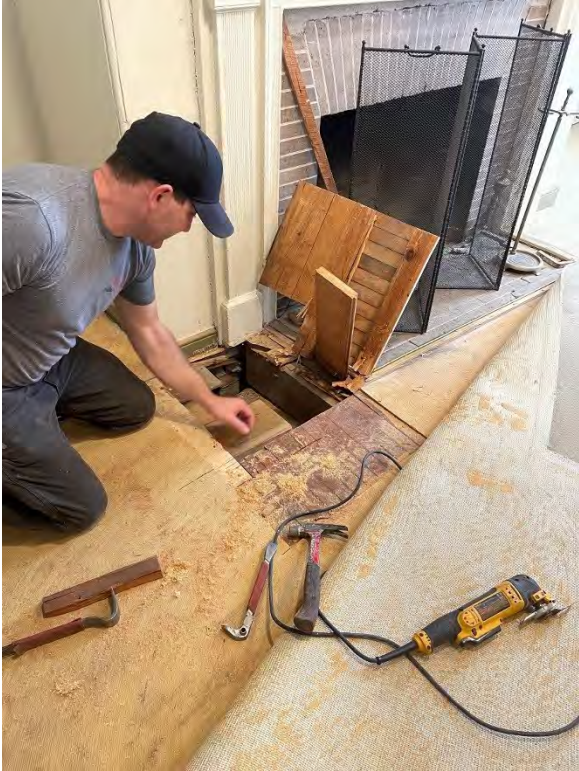
Photo I-29. Removal of flooring in southwest parlor to investigate the condition of the fireplace supports.
