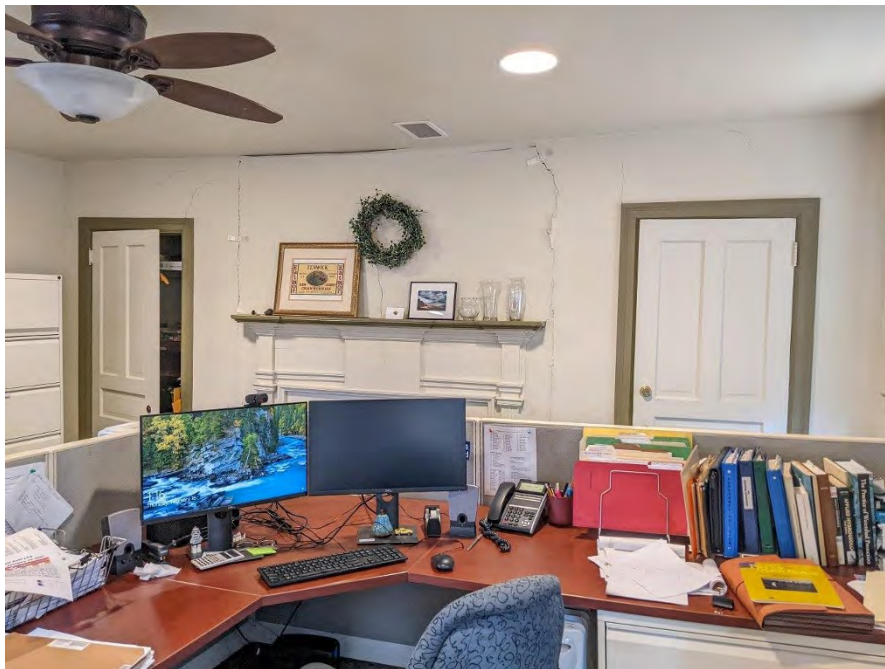
Photo I-22. View looking east within the former southwest bedroom. Note the cracking in the plaster around the fireplace.
