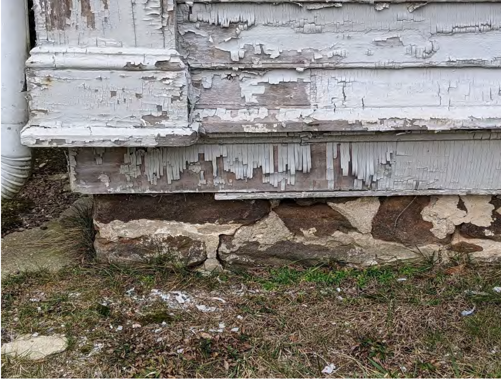
Photo E-21. View of mortar loss at the brownstone foundation. Foundations exhibit a mix of mortar and parging loss.
