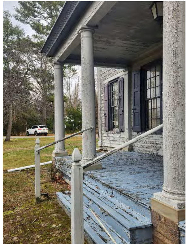
Photo E-10. Detail view of the front porch showing the Doric columns resting on limestone and brick piers. This image also shows the wholesale paint loss, which is throughout the painted porch elements.
