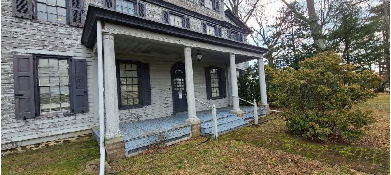
Photo S-1. View showing the front porch including the walk, which is barely visible due to the weeds and moss growth between the joints and on the surface of the brick. Note the grade is too high and there are two dead/dying bushes.
