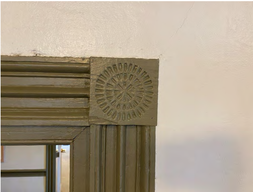
Photo I-14. Detailing of the corner blocks at the window and door surrounds in the western-most spaces.
