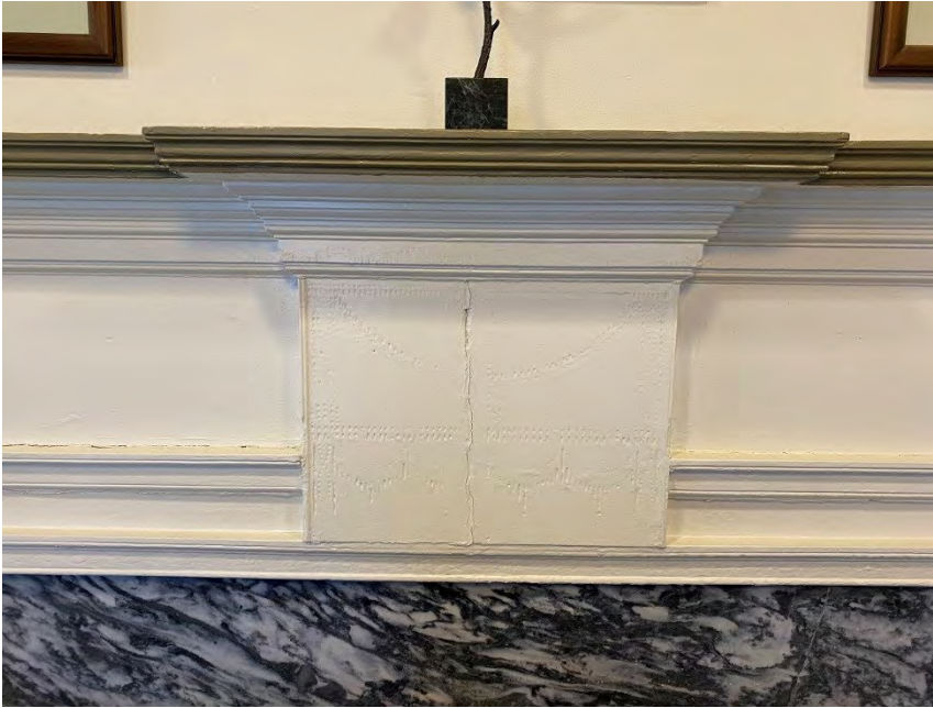
Photo I-35. Crack in the mantelpiece of the fireplace in the northwest parlor. There are conditions at this fireplace that indicate the supports here may also be undermined but not to the extent of the fireplace in the southwest parlor.
