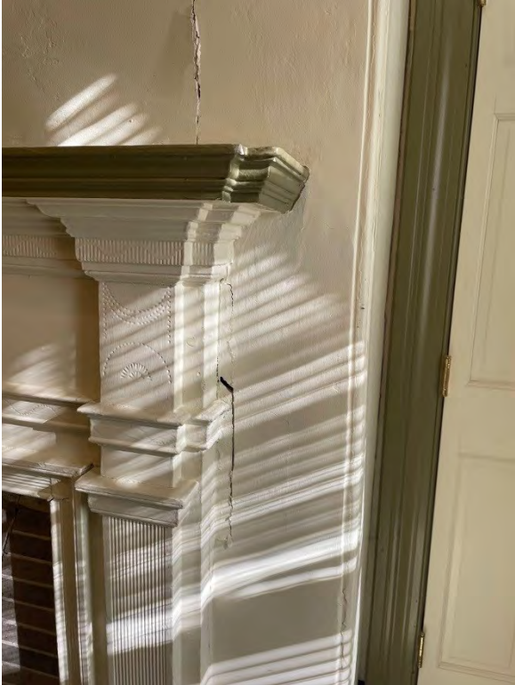
Photo I-33. Detail of the crack around the fireplace in the southwest parlor. Note also the detailing of the fireplace, which matches the treatment of the window and door surrounds.
