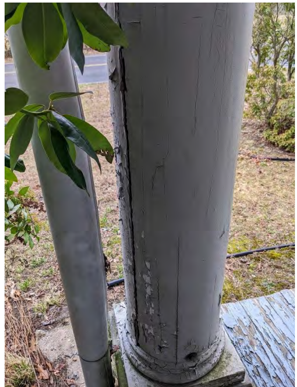
Photo E-22. Image shows a split in the south columns of the front porch.
