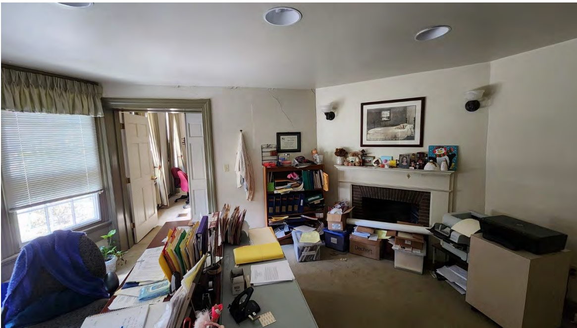
Photo I-16. View looking west at a first-floor office space and the corner fireplace, which would have been part of the first build of the Manor. The cracking adjacent to the corner fireplace is related to the issues with the fireplace in the southwest parlor.
