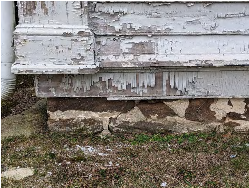
Photo E-14. Detail of paint that has checked, which is severe in many locations.
