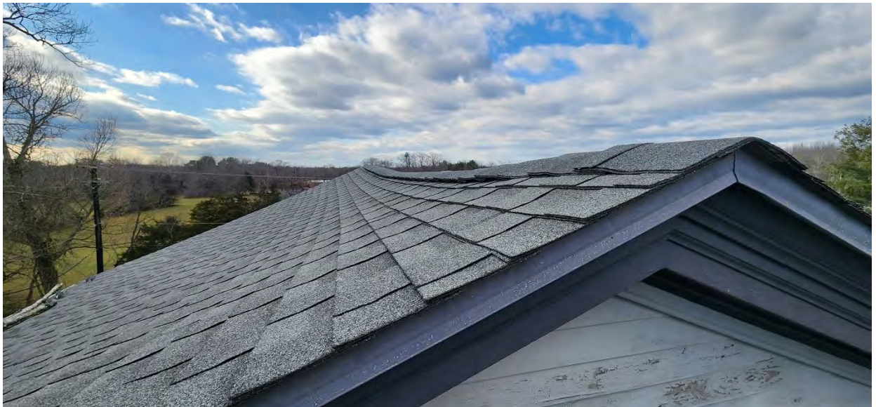
Photo E-26. This image shows a slight dip along the ridge of the west section.
