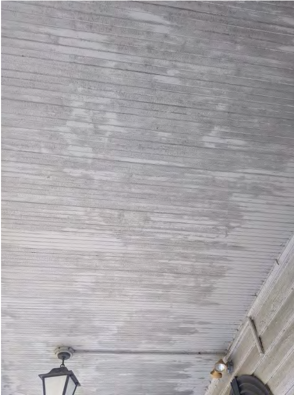
Photo E-19. Paint is alligatoring at the ceiling of the front porch.
