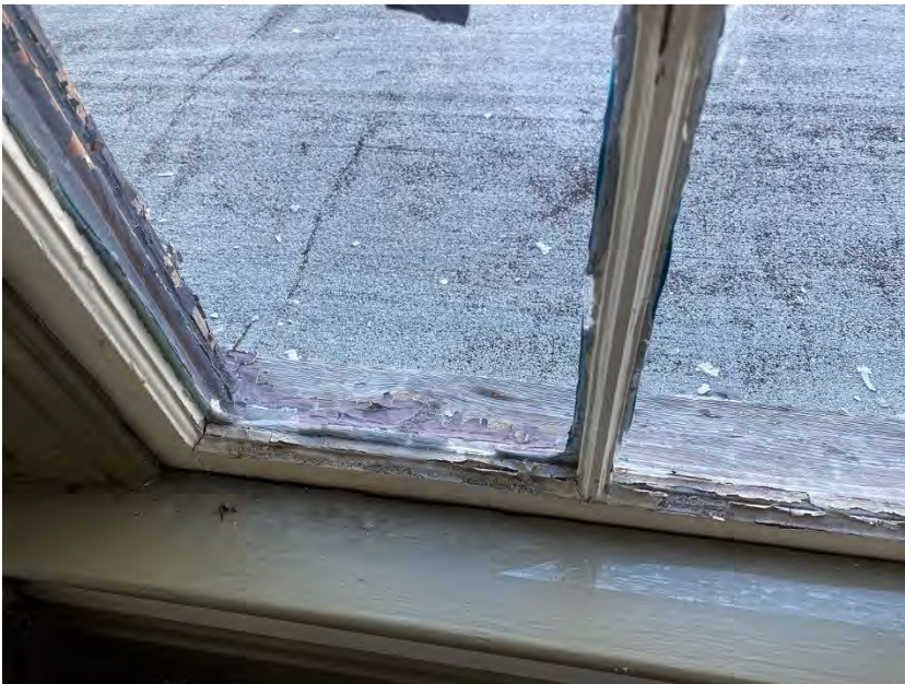
Photo I-38. View of a second floor window showing loss of paint at the exterior sills and the interior of the window sashes.
