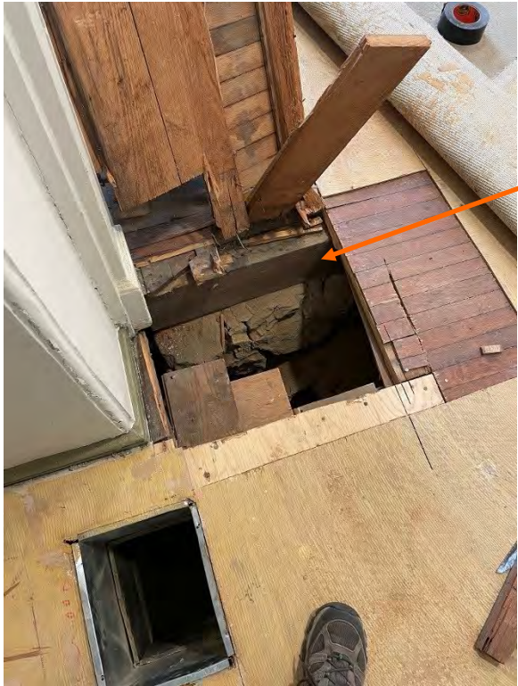
Photo I-31. Detail view of floor removed showing portion of foundation wall, which has been undermined by the digging out of the crawlspace of the HVAC ducts. Note the various layers of flooring under the existing carpet.
