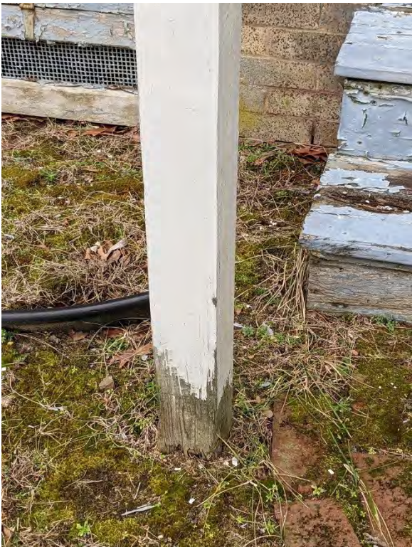
Photo S-6. Plastic edging indicates foundation plantings no longer present. The newel post for the railing at the front porch sits on grade and wood rot is evident at the lower few inches of the post.
