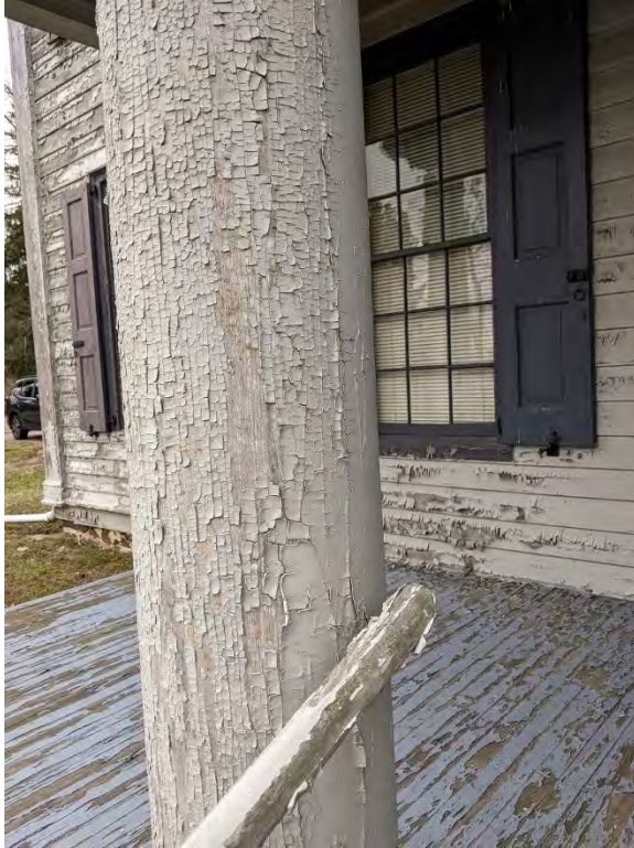
Photo E-13. Detail of alligatoring of the paint.
