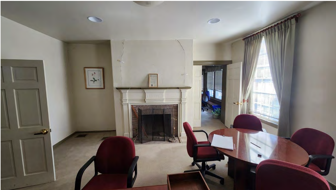
Photo I-12. View looking east at the southwest parlor. Note the cracking around the fireplace; there are other cracks along this entire wall and at the northeast corner of the space.
