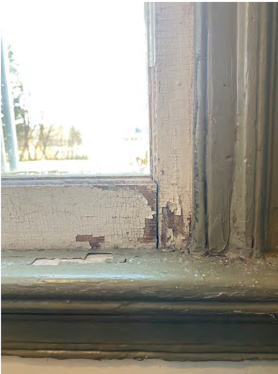
Photo I-34. Detail view of window sashes showing open joints, crazing paint on the sashes, and paint loss on the sills.
