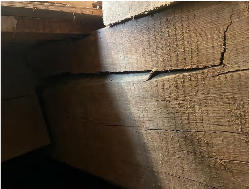
Photo I-30. View the cracked fireplace header, which supports three levels of brick masonry.
